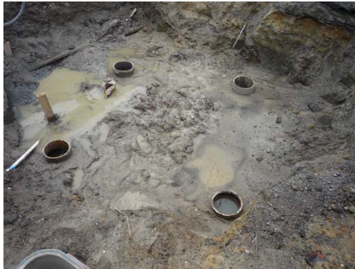
Signal Pole Footing Micropile Casings
