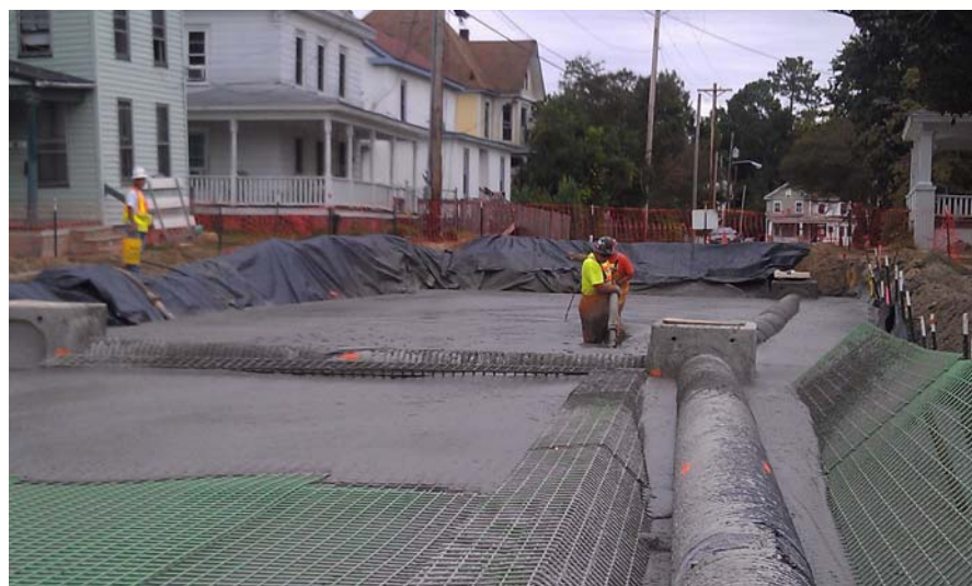
-Y- Line Foamed Concrete Placement
