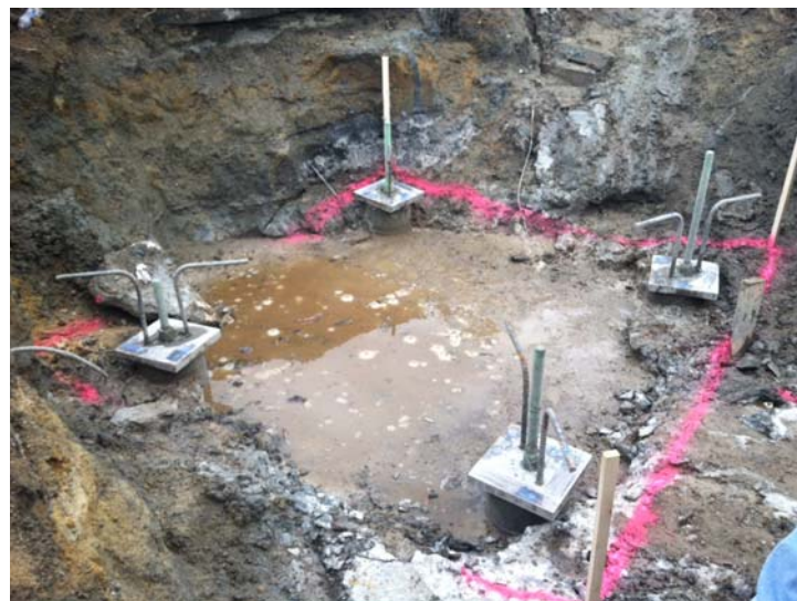
Signal Pole Footing Micropile Casings
