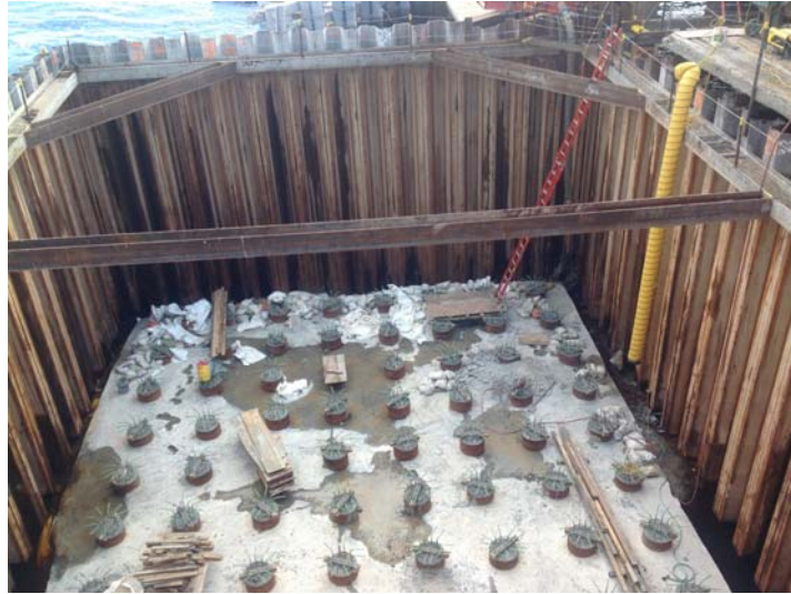
Pier 5 Permanent Foundation
