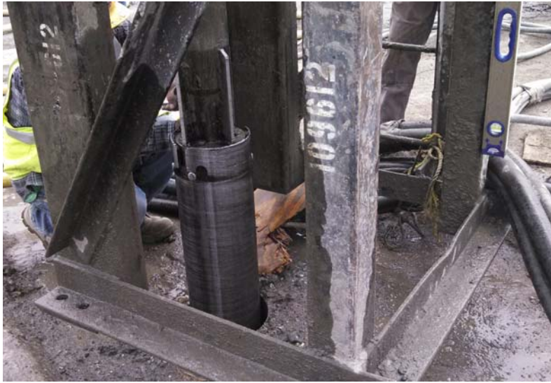
2 nd Micropile Drilling Technique, Bar Insertion after Grouting
