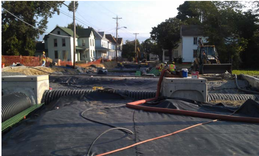
-Y- Line Undercut for Foamed Concrete
