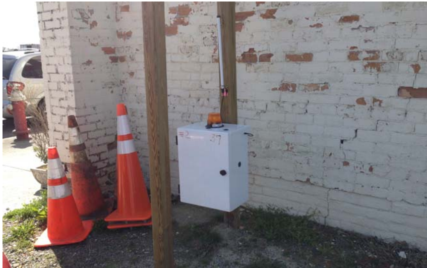
Permanent Vibration Monitoring Station
