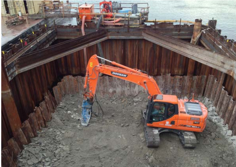
Pier 6 Existing Footing and Seal Removal
