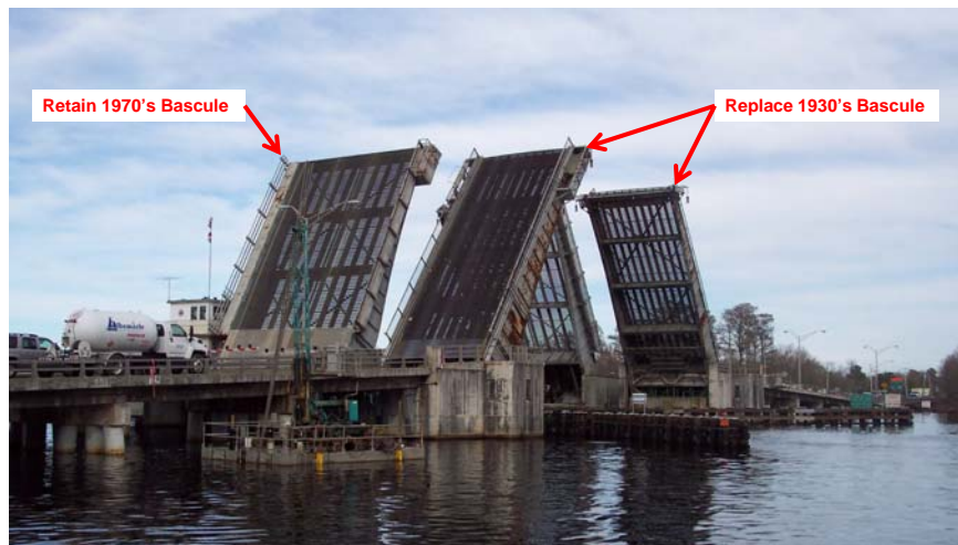
Removal and Replacement of 1930's Bascule Lift Piers
