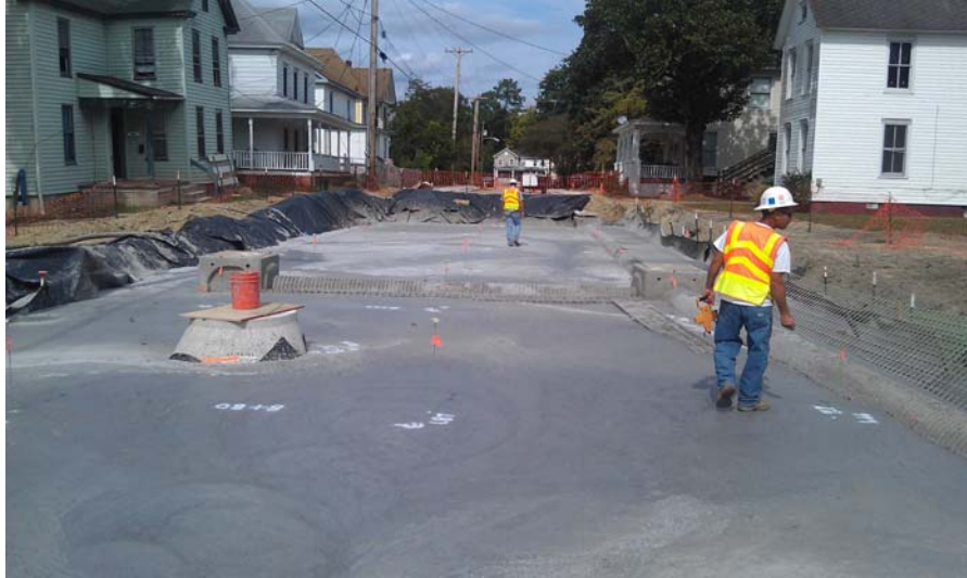
-Y- Line Foamed Concrete Placement
