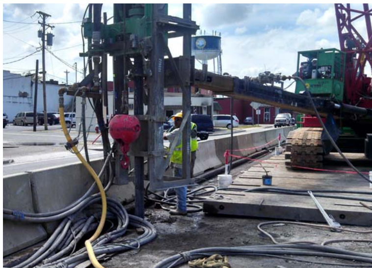
3 rd Micropile Drilling Technique, Insert bar through Drill Head
