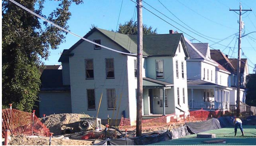
Pre-existing Building Settlement
