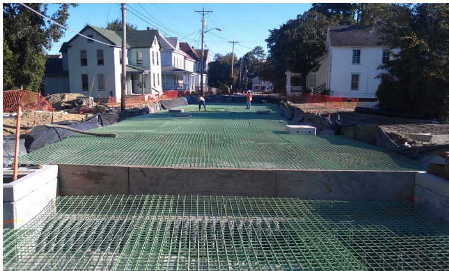
-Y- Line Foamed Concrete Placement
